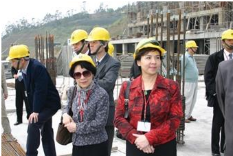
Dr. Flora Chang (right) accompanied Huang Pi-Twan, the president of TNUA and other visitors to inspect the construction progress of Lanyang Campus.
